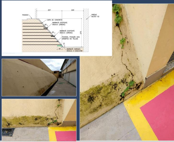
JGV Engenharia was called upon to carry out periodic verification of the containment structure of Fundação Bradesco in Salvador / BA. During our visit we noticed several cracks in the containment walls and accumulation of humidity in their base. With that, we recommended the correction of pathologies through the installation of new drains in the containment, in addition to cleaning and maintaining the existing drains.
