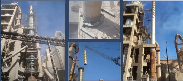
JGV Engenharia has partnered with Framar Engenharia to develop the structural reinforcement projects for a chimney, almost 100 meters high, which had been destabilized due to the high thermal loads that reduced the thickness of the chimney's metal plates, also aggravated by wind loads. The project developed urgently was conceived with metallic connections that made possible the displacement of the structure with the dynamic loads of wind and thermal.
