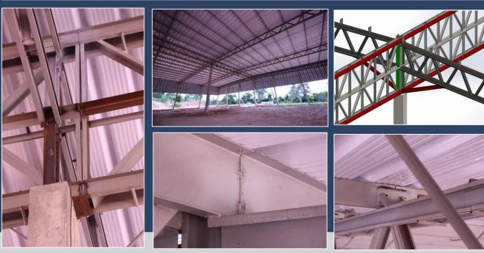
Structural Report and Structural Reinforcement Project developed for an industrial shed, where the roof and the metallic closure presented excessive displacements and torsions, caused by the incorrect design and dimensioning of the up to 40 meters long metal beams, a situation aggravated with the incorrect execution of the structure and oxidation spots.
