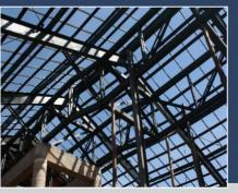
Due to dimensioning problems in the metal profiles, defective welds and loose connections, the metal structure partly gave way, before the assembly phase of the structure had even finished. JGV Engenharia was responsible for preparing the report and structural reinforcement projects for the roof, filling a span of 50 meters in metallic structure and ceramic tiles.
