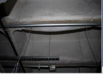
Technical Report and Structural Reinforcement Project for the installation of two safes at a branch of Banco Bradesco in São Paulo. We found that with the installation of the two safes, the ribbed slab would present displacements. JGV Engenharia developed the structural reinforcement project through sheets glued to the ribs, increasing the slab's load capacity in the section where the safes were installed.
